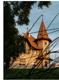
M.A.D House Exterior view
