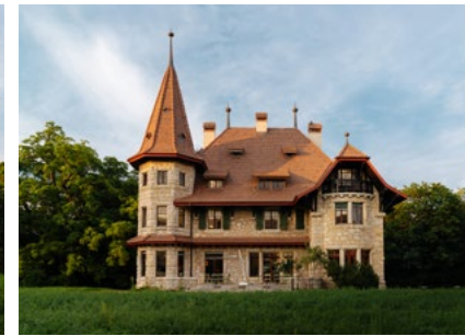
M.A.D House Exterior view
